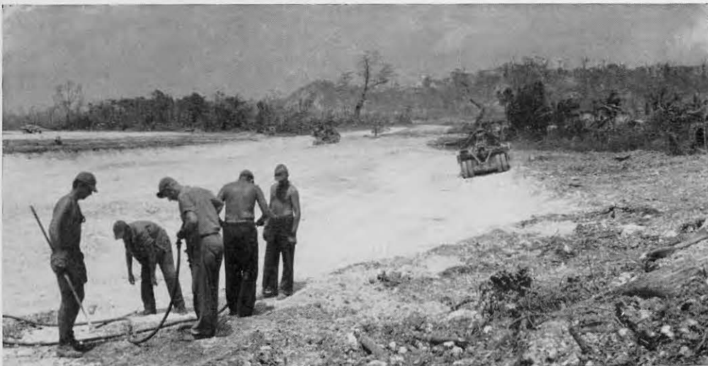
AIRFIELD PERIMETER ROAD
