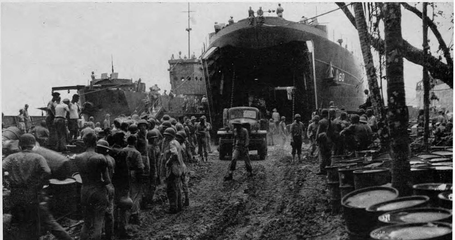
THE EQUIPMENT GOES ASHORE AT SASAVELE
