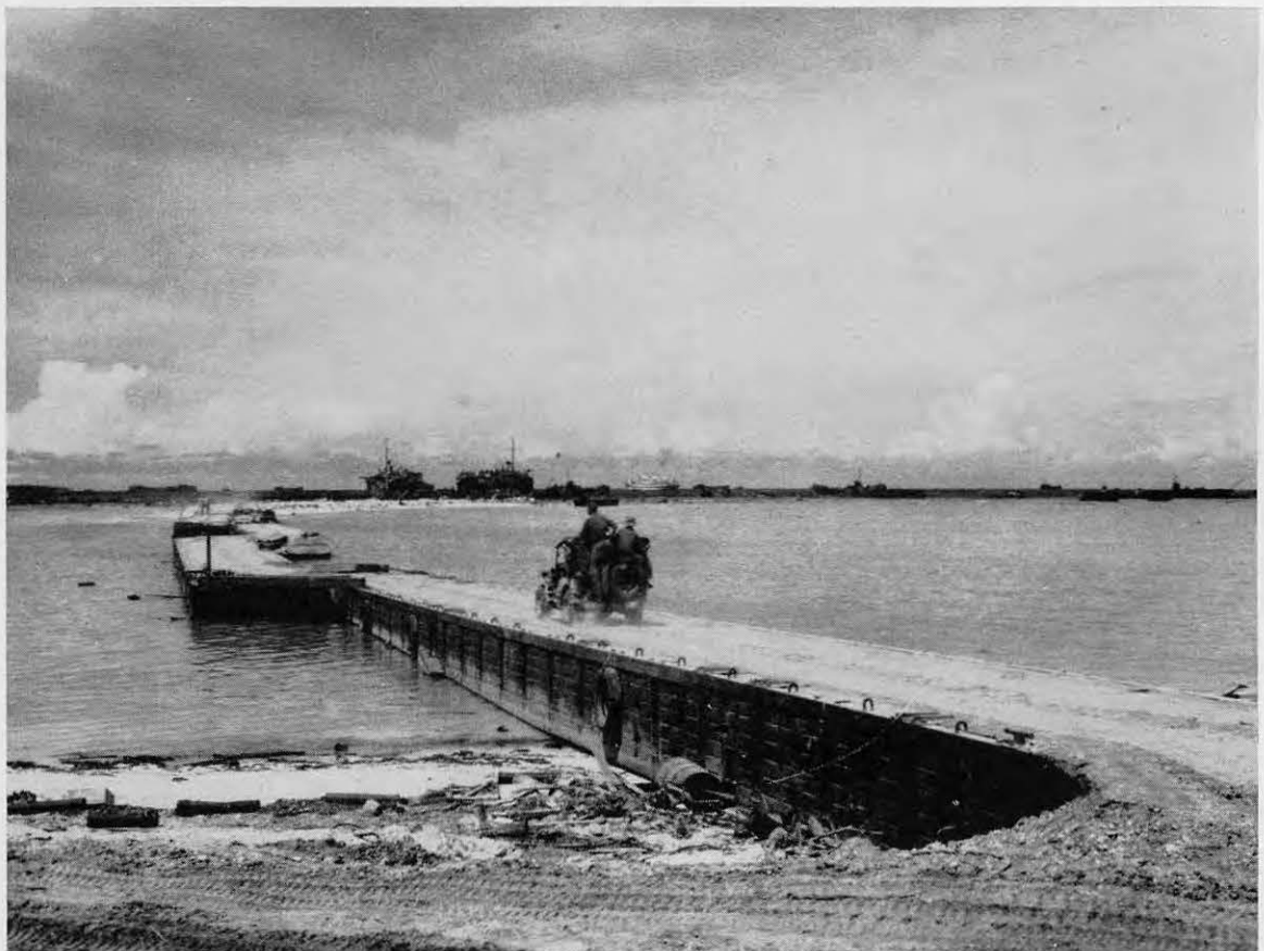
ORANGE BEACH PONTOON CAUSEWAY
