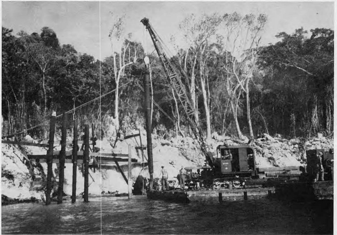
BUILDING PIER AT BAIRAKASERU
