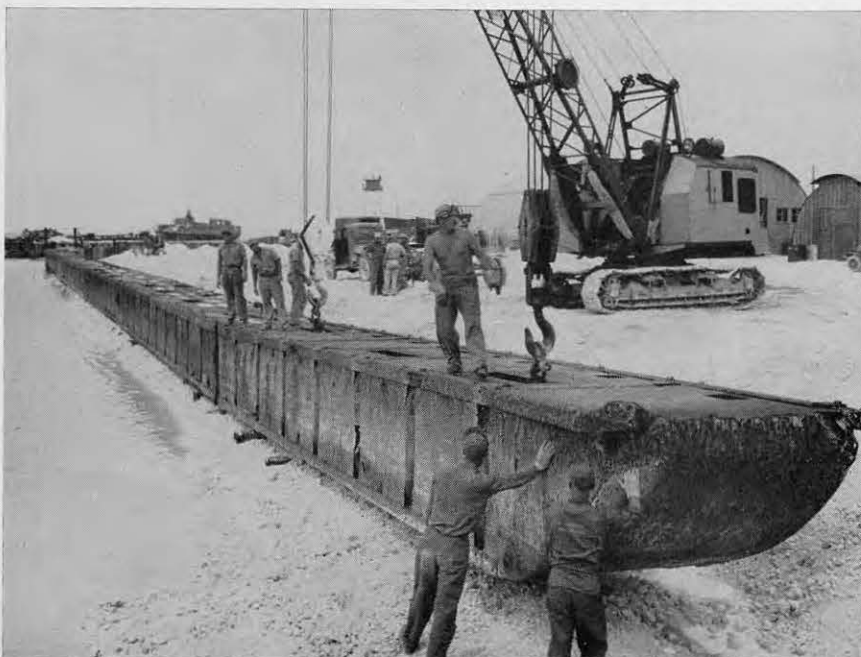
PONTOON SECTIONS LOWERED ONTO PILING TO FORM WHARF
