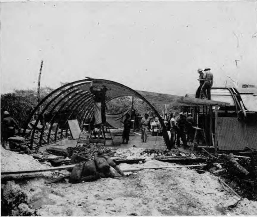
QUONSET HUT CONSTRUCTION
