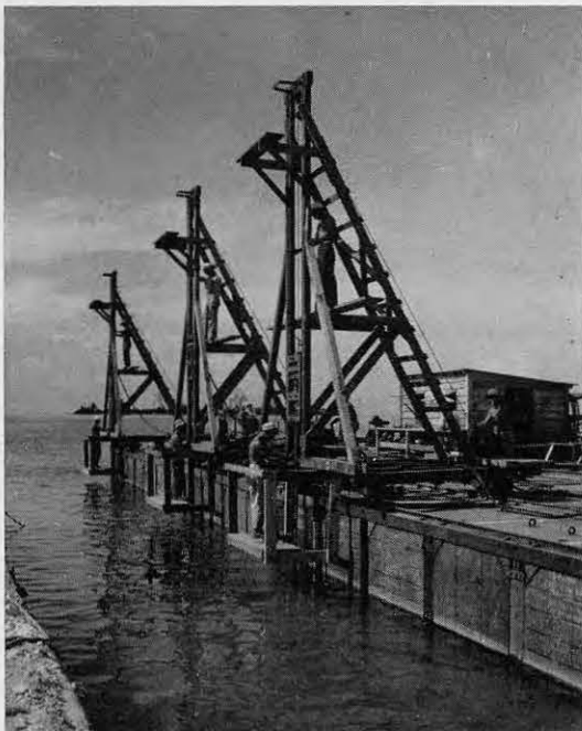
FIRST DRILL BARGE
