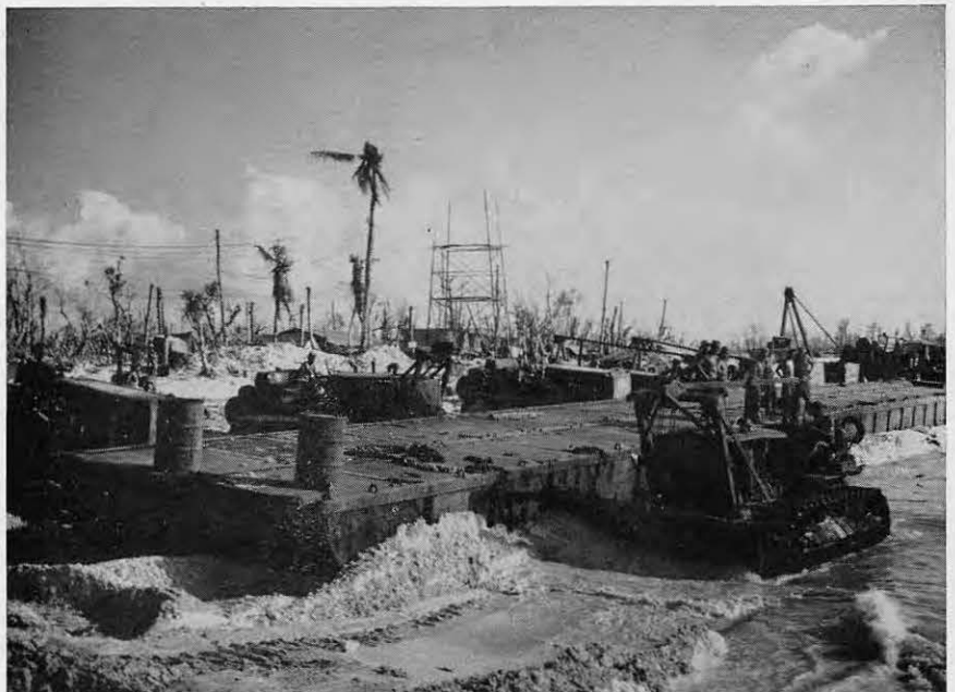
REFLOATING PONTOONS
