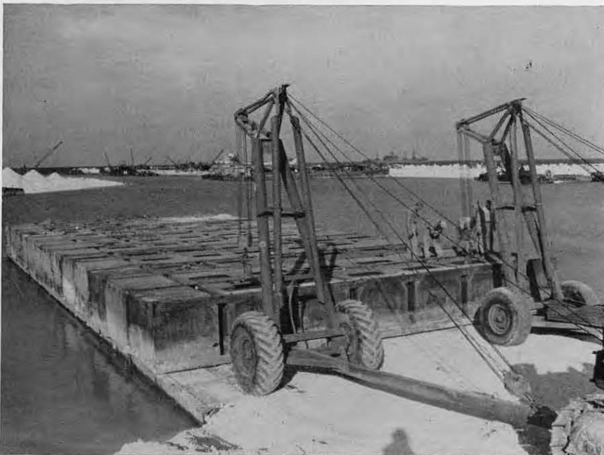
SETTING PONTOON SECTIONS FOR FINGER PIERS
