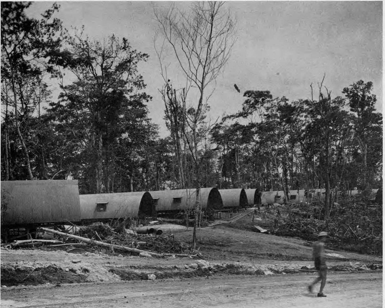
PILOTS QUARTERS NEARING COMPLETION
