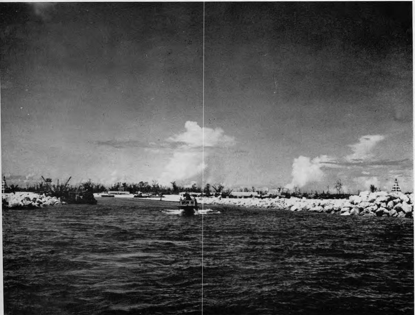
VIEW OF COMPLETED HARBOR TAKEN FROM SAME POINT
