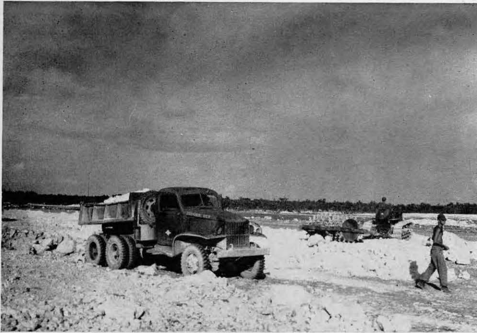
THE SUB-GRADING GOES IN
