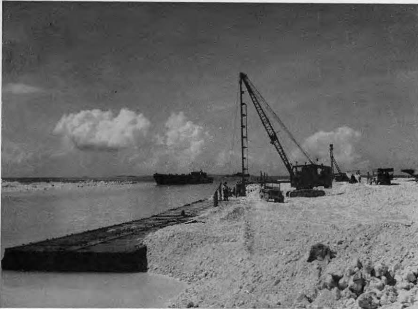
DRIVING PILING ALONG PONTOON WHARF
